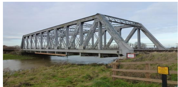
Figure 1.1: Truss Bridge Structure
