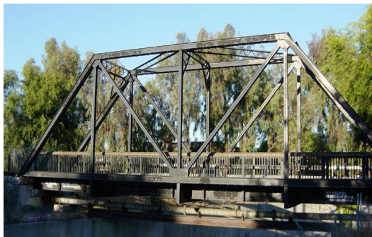
Fig. 1: Skeleton of a Typical Steel Truss Bridge
