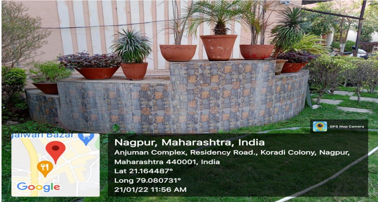
3) CONSEALED OPEN WELL (Besides first year building)
