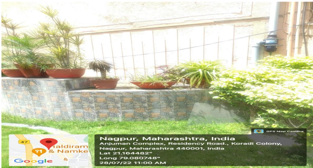
ROOF TOP RAIN WATER GET FILTERS BEFORE ITS TRANSIENT INTO OPEN WELL (From Roof Top of First year building)
